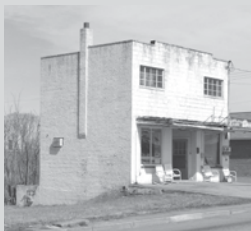
American Cab building 201 Fayette Street Photo by J. Siler
