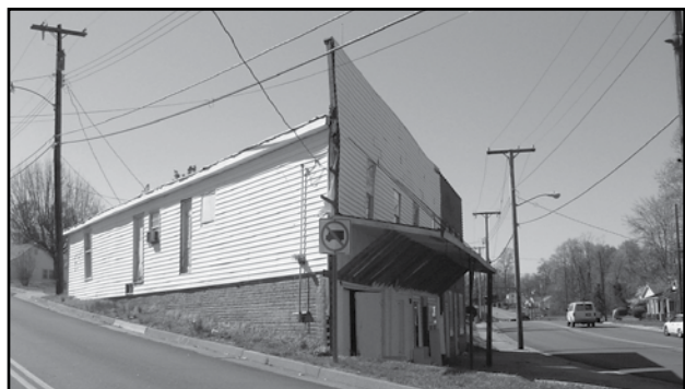
Former William D. Hobson Grocery, 1009 Fayette Street
